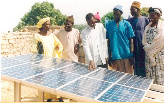
Solar panels to illuminate and operate house installations.
